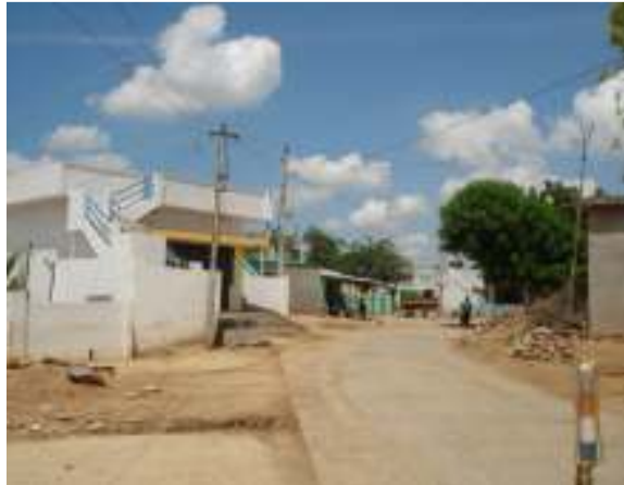
Photo 12: Water distribution networking location within Badvel town
